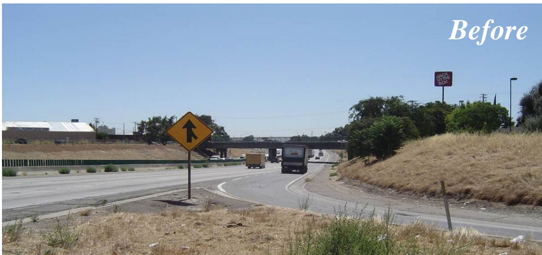
Viewshed #4: SR 99. Highway travelers' existing view from SR 99 looking south toward the Kansas Avenue overpass.
