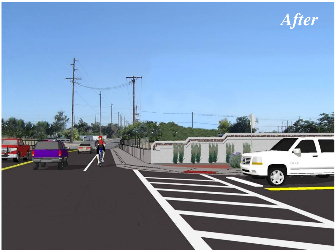
Viewshed #1: Rosemore Avenue. Simulated view of either build alternative at the completion of Phase 1. Note: The noise barrier on the right half of the simulation is no longer recommended; instead, there would be the same see-through railing-type barrier as shown on the overcrossing.
