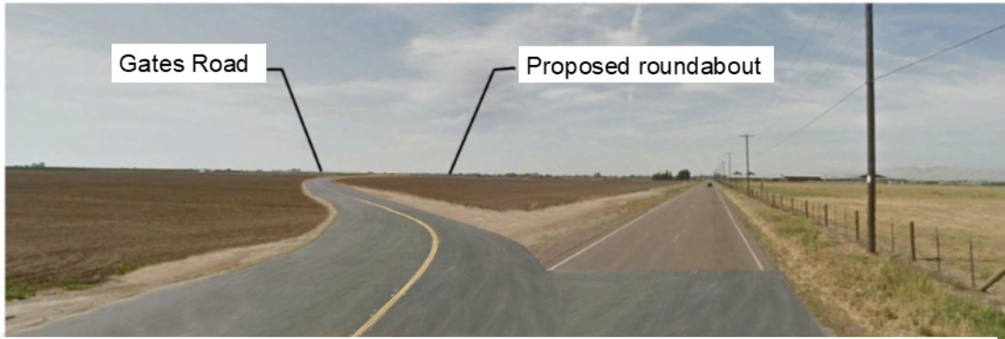
View looking southeast at realigned Gates Road toward roundabout.
