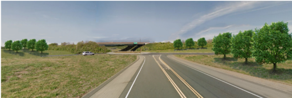
Proposed view looking north towards the spread diamond interchange and realigned Gates Road undercrossing for the new Alternative 2 alignment. Image shows possible agricultural themed landscape treatment.
