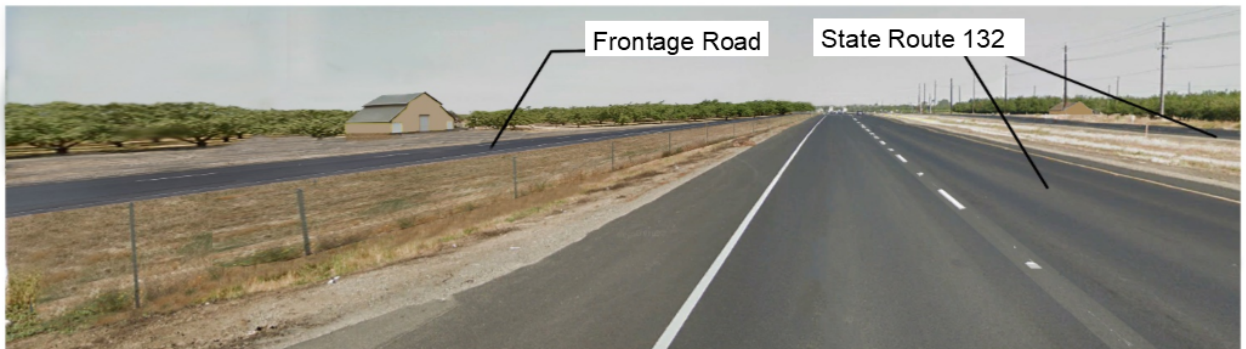
Typical frontage road adjacent to State Route 132 for Alternative 4 looking east.
