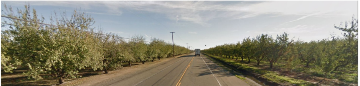
Existing condition State Route 132 looking east.
